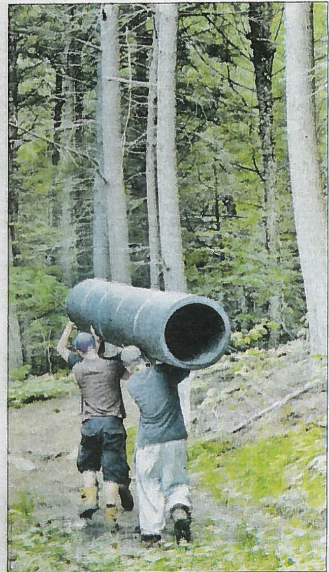
A gang of area Stewardship Rangers totes a drainage pipe through the pines and hemlocks of the LaCloche Ridge reserve as part of a trail maintenance assignment.
