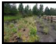
Graded slopes and native vegetation planted
