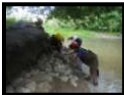
Ontario Rangers stabilizing a corner bank with cobble and boulders to prevent erosion
