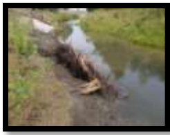
Root wads protecting the shoreline from erosion
