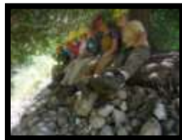
Ontario Rangers stabilizing a corner bank with cobble and boulders to prevent erosion
