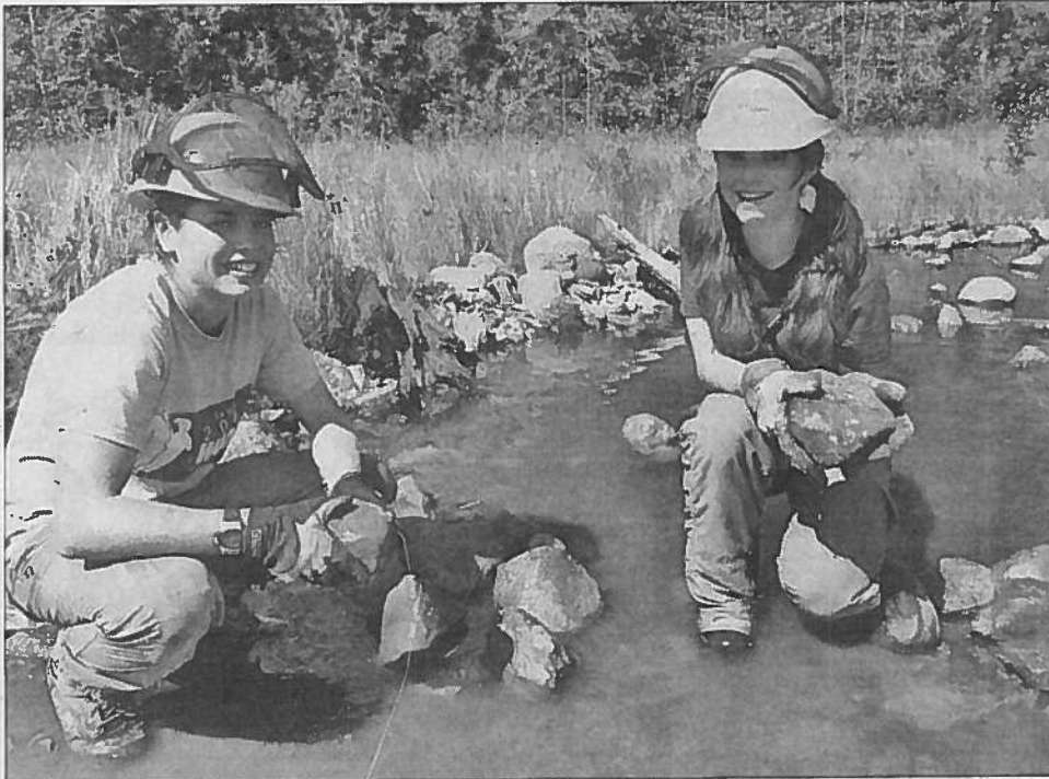
A stewardship ranger and her crew leader from Killarney Provincial Park construct rock weirs in Mill Creek near Meldrum Bay.
